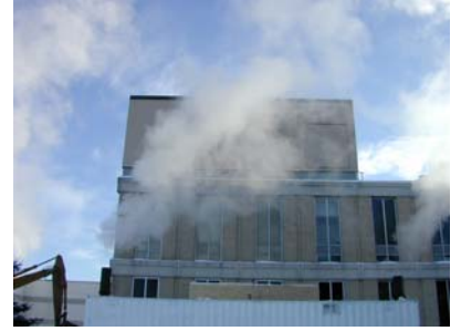
Mechanical Penthouse above sensitive areas.
